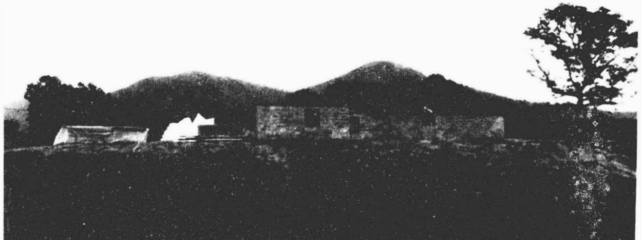
Site of the School looking at it from the West side. From this small
